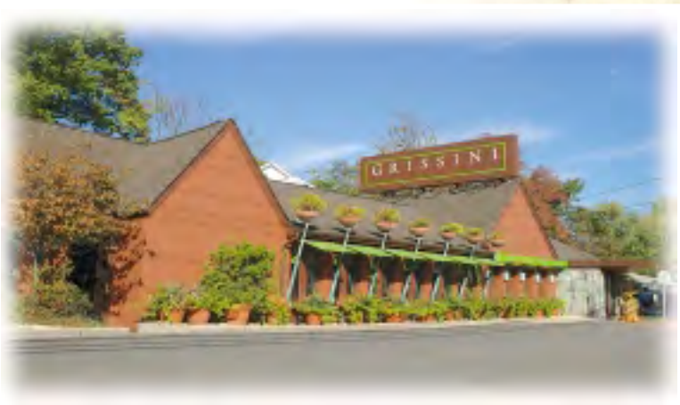
Grissini's Restaurant Englewood Cliffs, New Jersey
